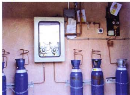
✓ Figure 1: Nitrous oxide manifold system
